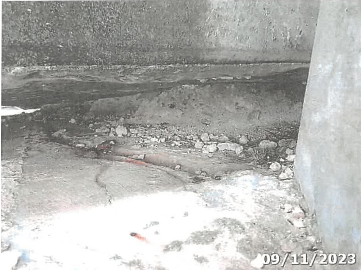
Photo 05 Element/Env 215/4: Re Conc Abutment
