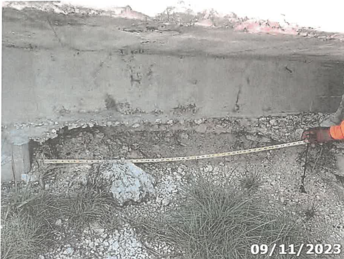
Photo 04 Element/Env 321/4: R/Conc Approach Slab
